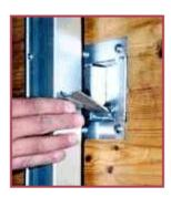
With the stall door in the closed position, set your gravity latch at the desired height and mark a 3" x 3 3/4" cutout area. (make certain the gravity latch can be reached from inside of the stall). Set the gravity latch so the stop is projecting out against the frame of the door, preventing the door from opening. Cut the opening as marked (approx. 3" x 3 3/4" with a recipricating saw.
