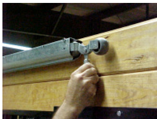
Upper Trolley Roller Bolt and Nuts Assembly Two Bolt and Nut Sets included in each hardware kit
