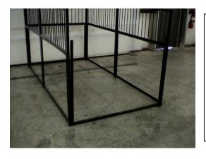
Install the back and side walls using the panel connectors and wall stiffeners as shown above before installing the bottom door frame. Insert the panel connectors on the bottom of the panel frames with the connector legs facing to the inside of the stall door frame.
