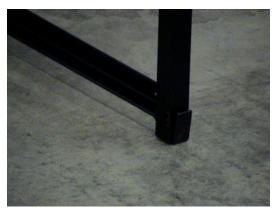
When seated correctly, the bottom panel connector will accept the bottom of the next modular panel.
