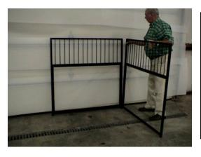
Position the next modular panel in place over the bottom panel connector in the first panel. IMPORTANT: If using a panel as a back wall, the side walls must be installed to the OUTSIDES of the back panel.
